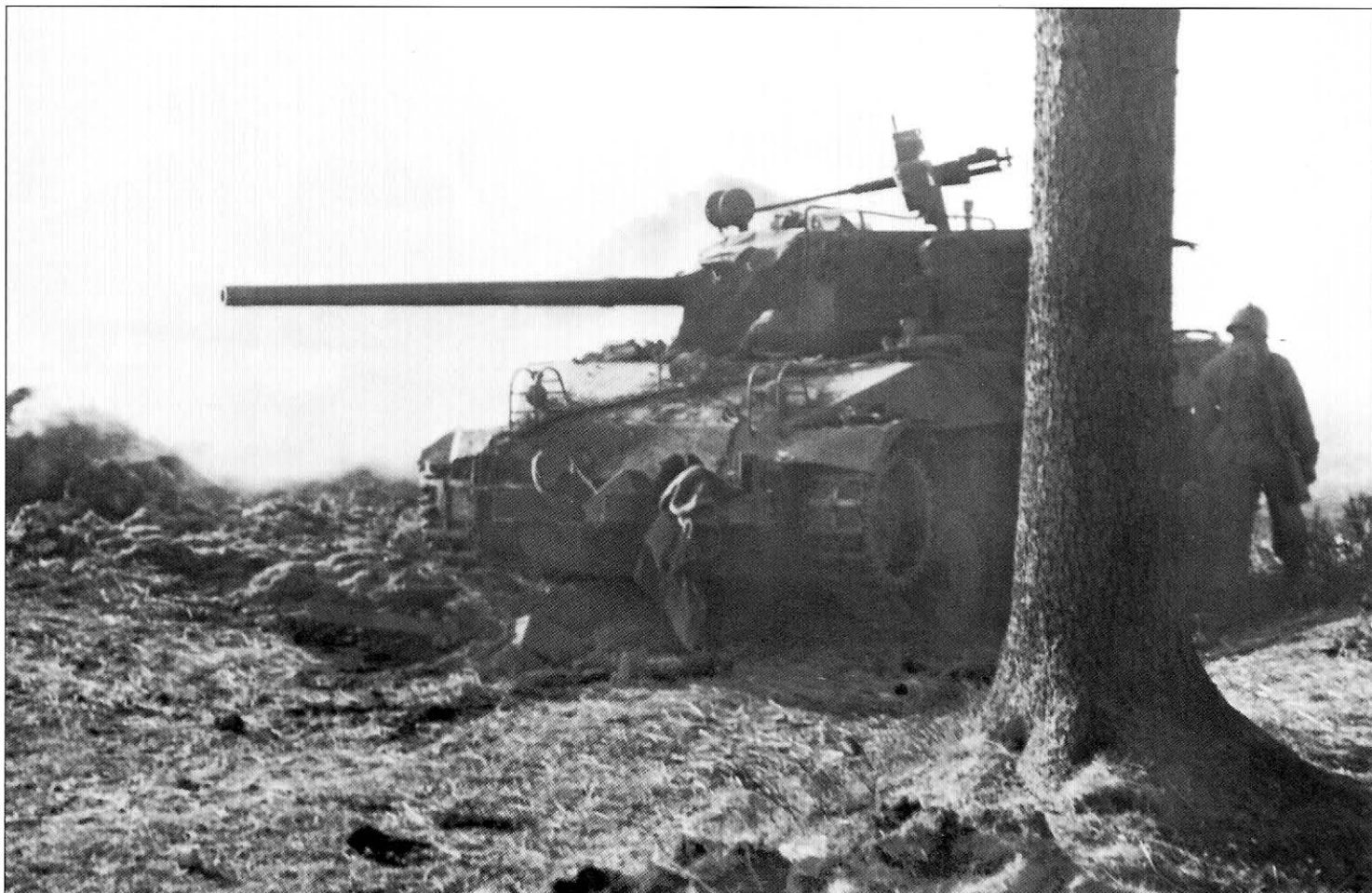
A 76mm Gun Motor Carriage M18, nicknamed the 'Hellcat', lies knocked out in field. The Hellcat was one of the best tank destroyer designs produced by the U.S. during the war and had a top speed of 55 miles per hour, almost 30 miles per hour faster than the other Sherman based designs. Its main drawback was its thin armor, not more than half an inch on most vertical surfaces, and the open top that provided little protection for its crew. This one appears to be a veteran of the Normandy battles judging by the Culin hedgerow cutters on the front.
