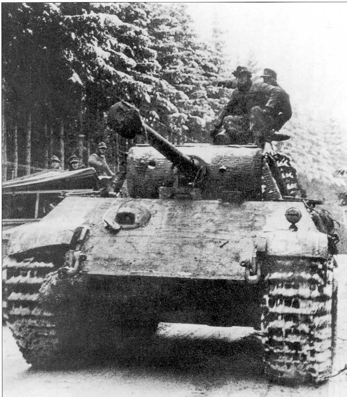
An early Panzerbefehlswagen Panther Ausf.G, still carrying its Zimmerit coating, passes a column of Schwerer Wehrmacht Schlepper half-tracked transport vehicles on a tree lined forest road. The outline of the star antenna can just be seen to the right of the commander, mounted in the normal vehicle radio antenna mount on the left side of the engine deck.
