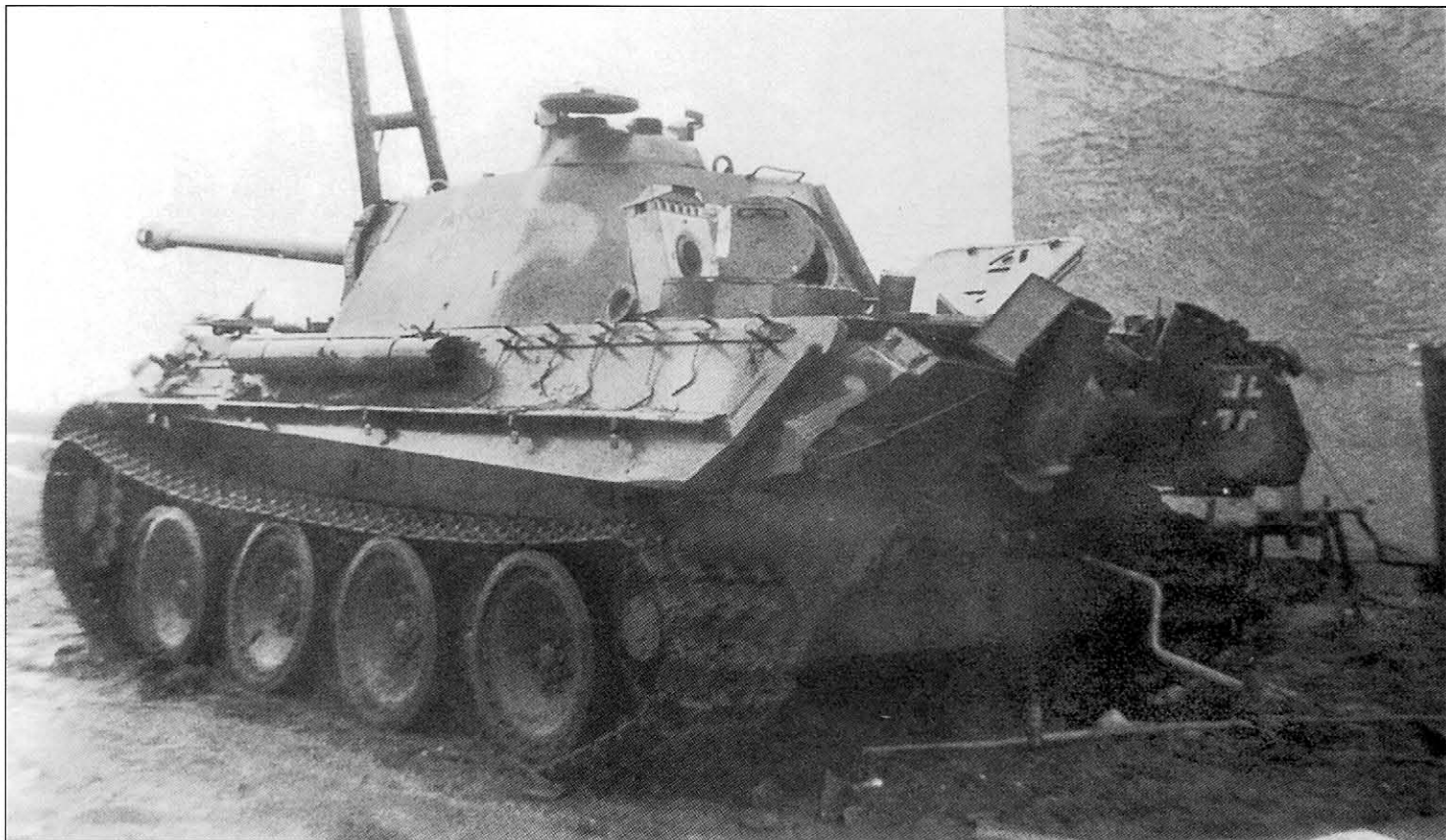
A new Panther Ausf.G, possibly from 9.Panzer-Division, sits abandoned in Clervaux, Luxembourg, the victim of a mechanical breakdown. This late production vehicle is fitted with the chin mantlet, Flammvernichter flame suppressing exhausts, raised fan cover for the crew compartment heater and new, larger diameter self-cleaning cast idler wheels. The three digit tactical number '301' is painted in a white stenciled outline on the sides of the turret and in solid white on the rear of the turret.
