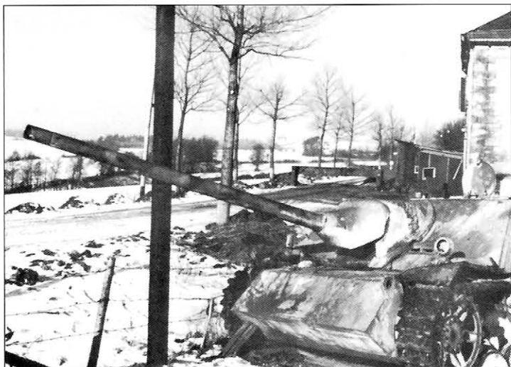
A Jagdpanzer IV/70 (V), probably from SS-Pz.Jg.Abt.1, sits beside the Bastogne-Wiltz highway on the border between Belgium and Luxembourg. This is a late production vehicle with resilient steel wheels on the front two stations and three steel return rollers. The gun travel lock, normally fitted to the glacis plate, appears to have been torn away. Remnants of an 'ambush' camouflage scheme can be seen on the upper fighting compartment and open hatch.
